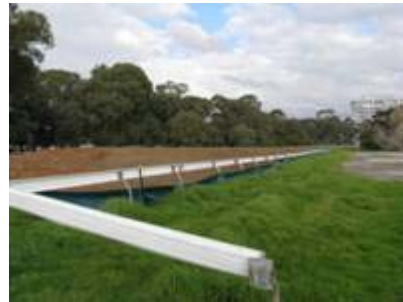
Temporary soil storage
